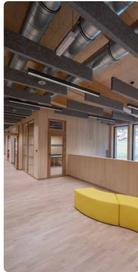
Secondary School Matrei, Austria Photo: Joachim Rauch
