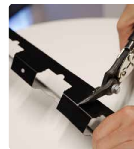
Flexible on-site adjustment is possible, allowing the rail to be easily cut with metal shears.
